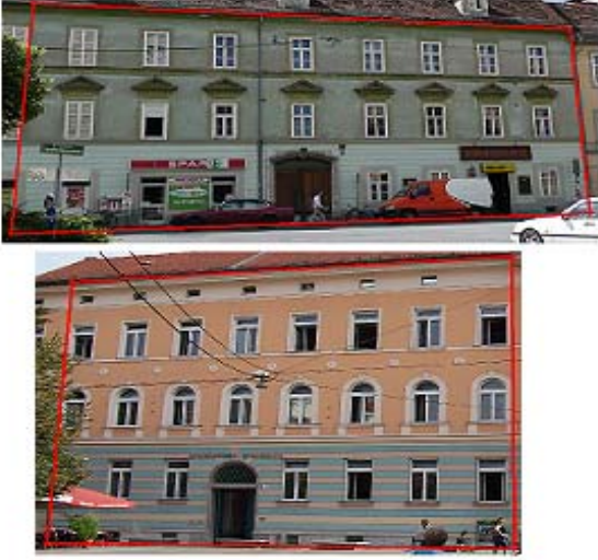
Figure 2: k-means clustering in CIE-Lab color space. Top row – façade with uniform color and its clustering visualization on the right side. The façade in the bottom row consist of areas with several different colors. This non-uniformity express by itself as several different clusters in a color space.
